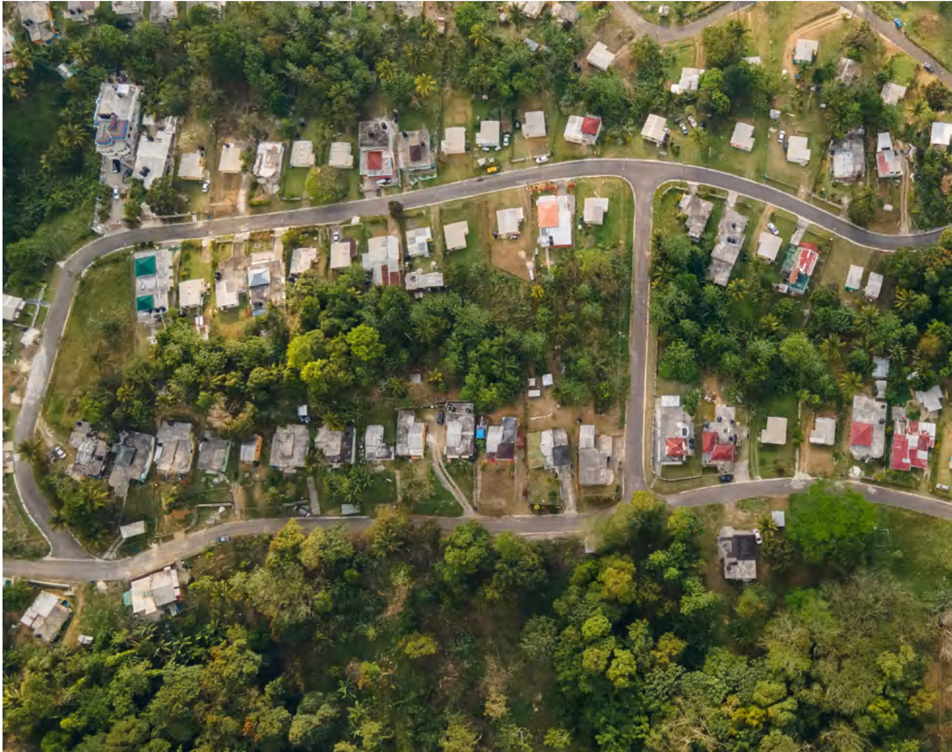
Bethel Town Housing Scheme - Aerial View, Westmoreland
